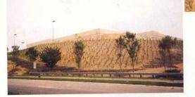
planned solution of over-excavation and riprap fill.
